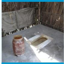
Space: An accessible toilet has enough space and light. The floor is not slippery & is easy to clean.
