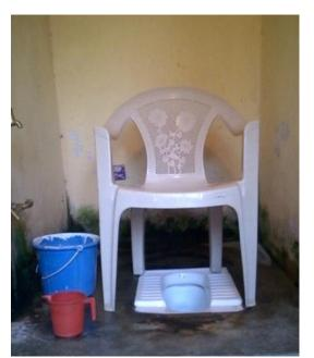
Cut a central hole from a plastic chair and smooth down the edges A simple toilet seat can be constructed by adapting a plastic chair and cutting a hole in the centre. Be sure the cut edge is smoothed.
